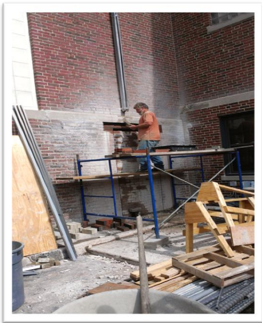
Masonry work on pool exit.
